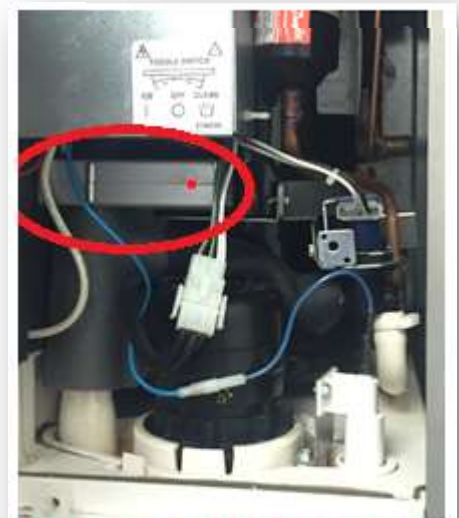
HydroFLOW Installs on the Circulating Water Line
