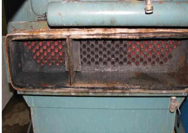
Heavy corrosion has been removed from steel and a protective dark gray layer of magnetite is beginning to form
